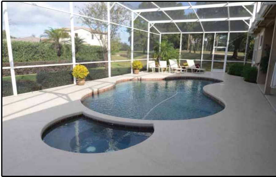
Screened Enclosed Pool
