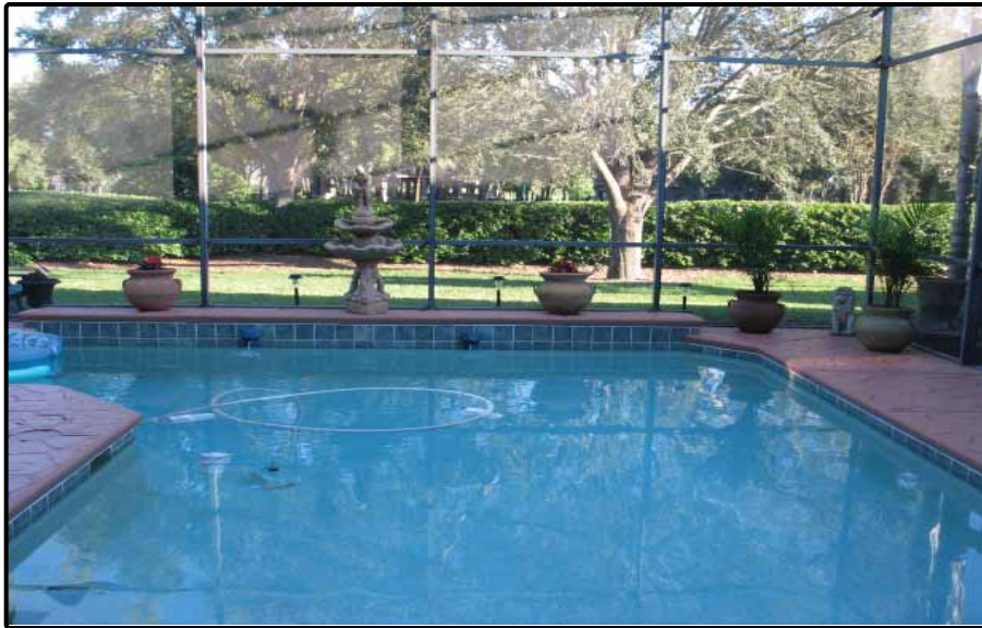
Screen Enclosed Solar Heated Pool
